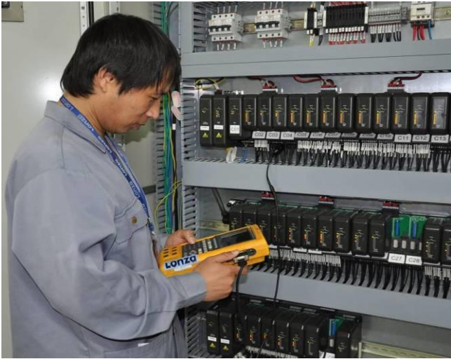
Instrument I/O loop test
